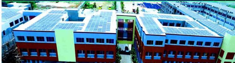
500 kWp Roof top Solar Plant
